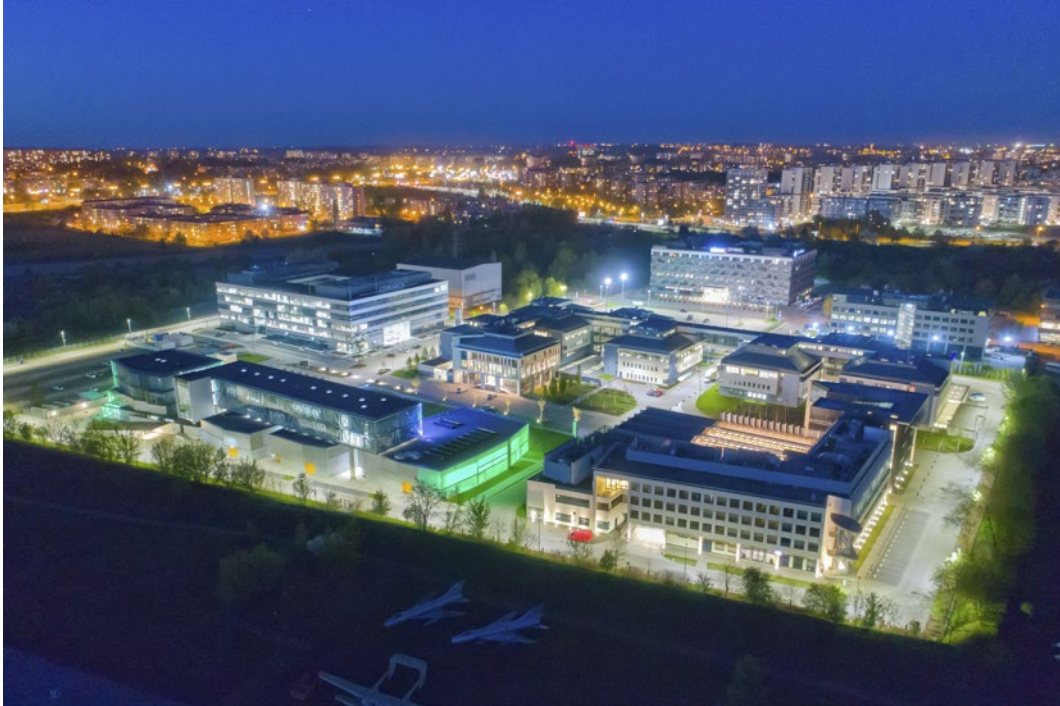
Comarch headquarters in Kraków
